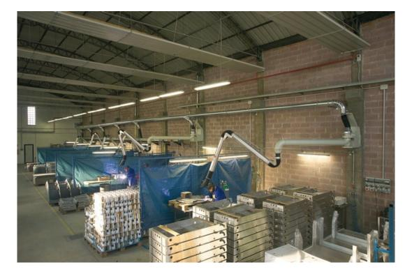
The extraction arms are suitable for extraction of fumes at temperatures of up to 280°C due to the use of 304 AISI stainless steel and flexible couplings in dual-layer double silicone fabric. The capture hood is made of sheet metal and coated black to prevent irritating light reflections.
