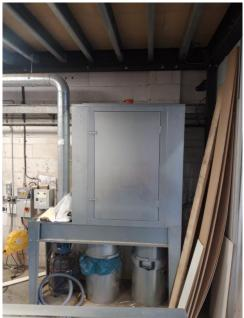
The above example is of a turnkey installation of an LEV system to a table saw and chop saw. Our in house electrician is able to complete all wiring to take the hassle away from you.
