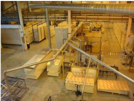
Our solution was to redesign the factory ducting layout to ensure efficient extraction to all areas. In particular the range in ducting sizes varied from 840mm diameter at the extraction unit to 80mm diameter at source.
