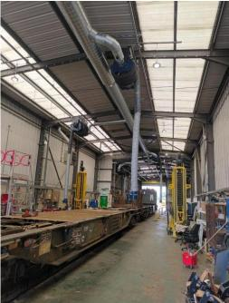
Even though engine standards become ever more stringent, extraction systems are still required to remove harmful exhaust fumes and protect persons in an enclosed space.
