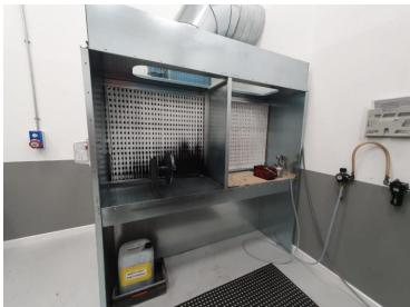
An internal fan set was installed which then exited the building and expelled fumes above the roofline safely to atmosphere via a high velocity jet cowl.
