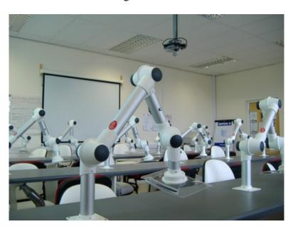
A total of 18 aluminium extraction arms were installed in the classroom each terminating with extraction hoods to ensure complete extraction of fume. The fume then passes through an activated carbon filter which enables the cleaned air to be expelled to atmosphere.
