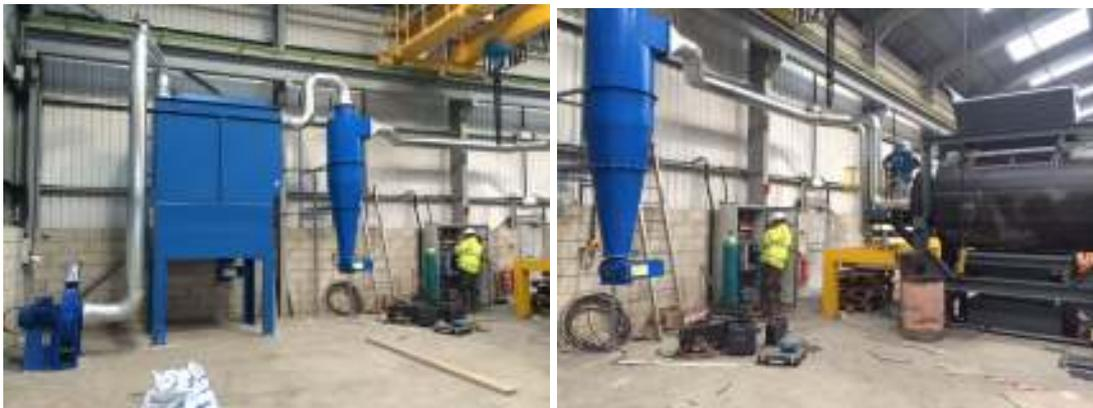
Due to expansion of the process an additional cyclone has been fitted to the extraction system by ourselves.
