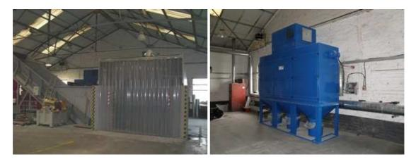
The chamber was ducted to an ATEX filter unit which is capable of extracting an air volume of 9,250m<sup>3</sup>/hour. The units three dust storage bins each have a 100 litre capacity and are quick and easy to empty.
