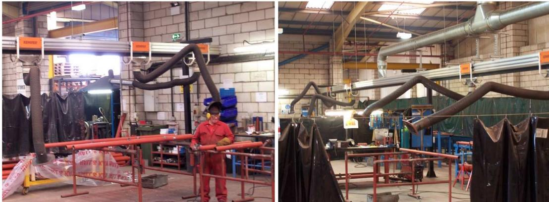
Extraction Rails are an advantage when working over a huge workspace on large items. Each exhaust arm is attached at a height of three metres and is rotatable through 360° due to its positioning on the rail. This gives the operator a free and unobstructed working area. In addition the arms are able to be moved to any point along the rail giving this workshop a floor area of 360m<sup>2</sup> covered by extraction.
