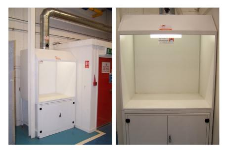
The booth exceeded the client's requirements and was able to be fitted in a tight corner on the shop floor. In addition to providing fume extraction where operatives mixed paint, the booth was internally illuminated for ease of use.
