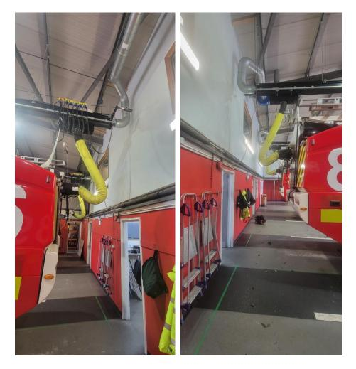
Even though engine standards become ever more stringent, extraction systems are still required to remove harmful exhaust fumes and protect persons in an enclosed space.
