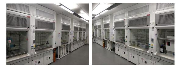
In total 24 Fume Cupboards were installed with appropriate storage. In addition PVC ducting was used to transport the chemical fumes to an appropriate polypropylene centrifugal fan. The fan was housed on the roof and then vented to atmosphere to safely disperse the contaminant.
