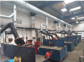
The twelve workstations each have a two metre long extraction arm and hood that are both rotatable through  $360^{\circ}$  to ensure workers are covered at all times during all welding scenarios.
